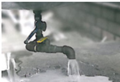
Untreated compressed air does not prevent large amounts of water from collecting in air receivers and downstream piping.
